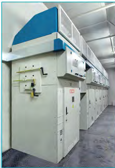
1S-UZSSP-3.3 Semiconductor grouping point module with protection device panel for splicing station.
