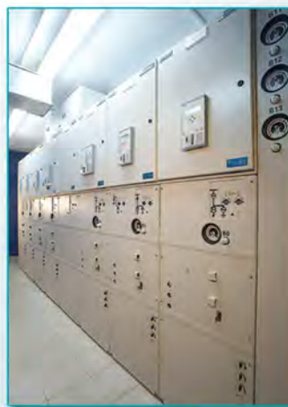
Medium voltage AC switchgear 35 kV functional unit One-side access, indoor installation, panels K-201 series or similar. Nominal current up to 2500 A, up to 6 panels per unit.
