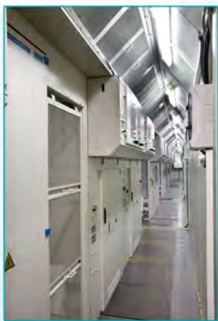
Medium voltage AC switchgear 2x25 kV functional unit One-side access, indoor installation, panels 1S-2x25, K-200 series or similar. Nominal current up to 1250 A, up to 3 panels per unit.
