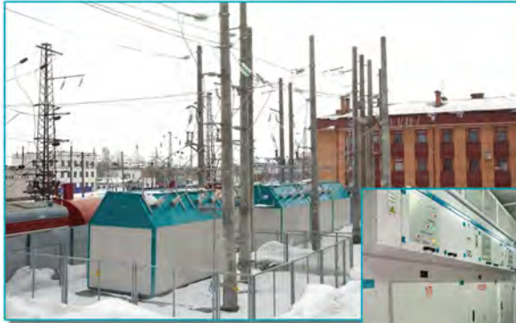
Modular type grouping point PG-M-3.3/27.5
