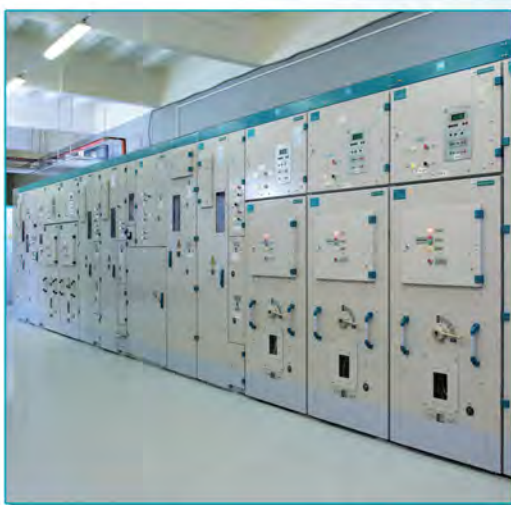
Medium voltage DC switchgear 3.3 kV functional unit One-side access, indoor installation, panels KV-3.3 series or similar. Nominal current up to 6300 A, up to 4 panels per unit.
