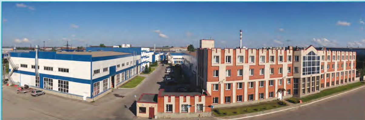
Administration and engineering buildings of NIEFA-ENERGO
