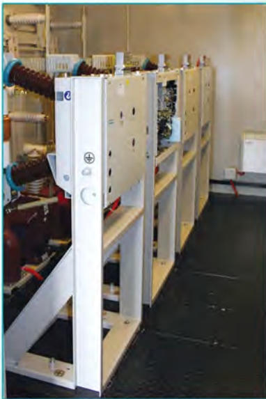
The high-voltage compartment of AC sectioning point PSK-25-2
